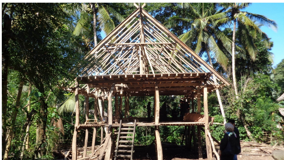
Figure 8. Frame of an Ammatoan house
