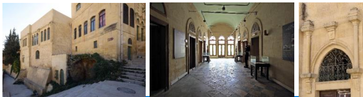
Figure 12. Different Views from As-Salt City historic buildings within the Golden era [4635].
